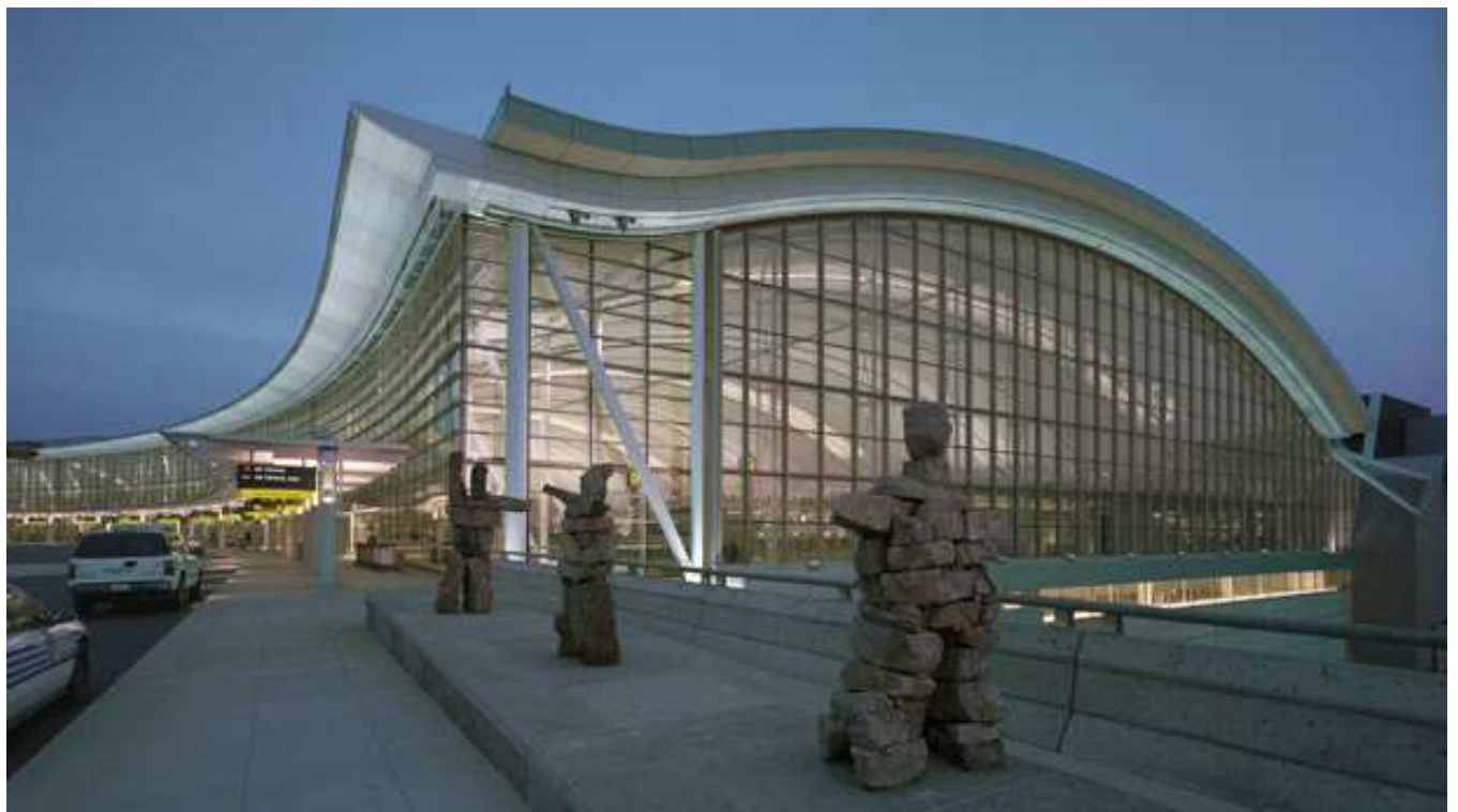
Figure 10-1: There are over 420,000 employment opportunities in Mississauga providing jobs for local as well as regional residents. While the largest concentration of these employment opportunities is in the northeast quadrant of the city at the Airport and surrounding lands, Mississauga has a number of other thriving employment areas. Mississauga has been highly successful in attracting office employment and over the last 25 years the city has developed an average of approximately one million square feet of office space annually. (Robert Speck Parkway Business Area, Hewlett-Packard Building, Airport -Terminal 1)
