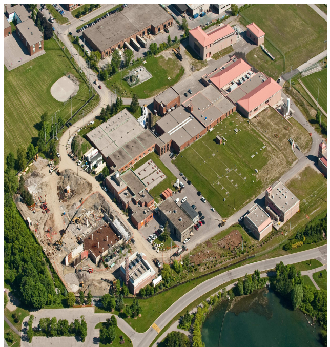
Figure 10-8: The 27 hectare Lakeview Water Treatment Facility is located on the shore of Lake Ontario in Mississauga and is operated by the Region. The Region has identified the need for a capacity expansion of the facility as a result of increased growth to serve the eastern part of Peel and to meet servicing requirements in York Region. The expansion of the Lakeview plant will increase capacity to produce 1 150 million litres of water per day.
