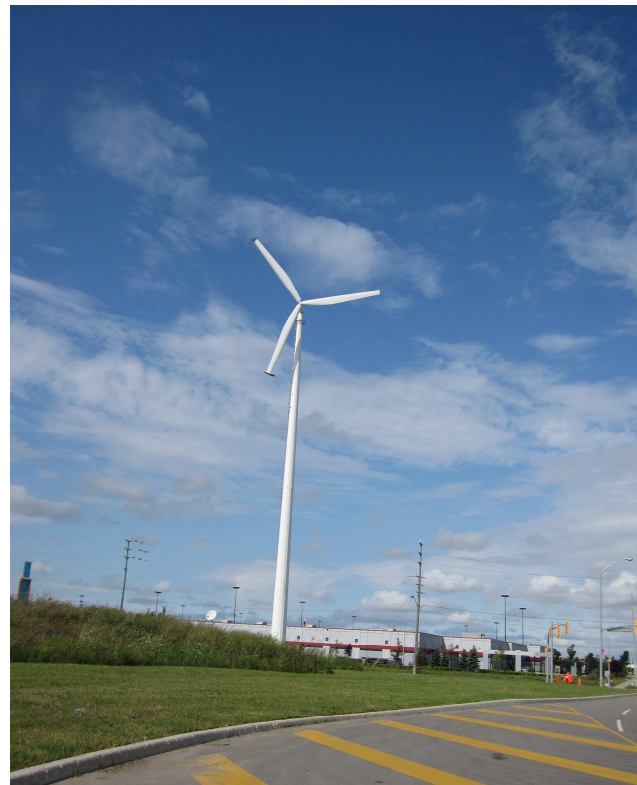
Figure 10-11: A 31 m wind turbine unveiled at the Lisgar GO Station in April 2009, generates as much as 80 per cent of the station's power. The site, located at Tenth Line and Argentia Road, was chosen for the wind turbine because of heavy prevailing winds from the west and its open fields.
